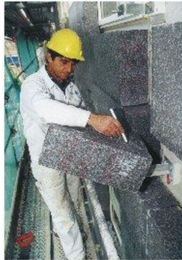
Figure 4.84 BASF retrofit (a) installation of external insulation, (b) installation of plaster with micro-encapsulated phase change materials
