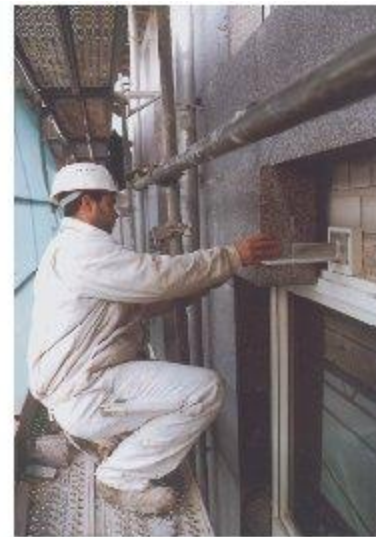
Figure 4.84 BASF retrofit (a) installation of external insulation, (b) installation of plaster with micro-encapsulated phase change materials
