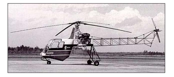
Eng. B.Sznycer, a graduate of the Warsaw University of Technology and a former employee of LOT Polish Airlines patented the "Omega" helicopter - the world's first flying crane (BS 12D). His patent (US No. 2,973,923) was used by Sikorsky Helicopters Corp., which created the S-64 Skycrane - giant helicopter with a payload up to 10,000 kg.
